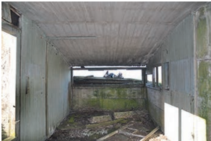
Figure 11.25 The western observation room of the former Fire Command (North) (© Gordon Barclay)
