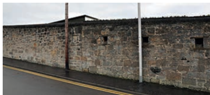
Figure 11.73 Surviving portion of the loop-holed boundary wall on Pettycur Road (© Gordon Barclay)
