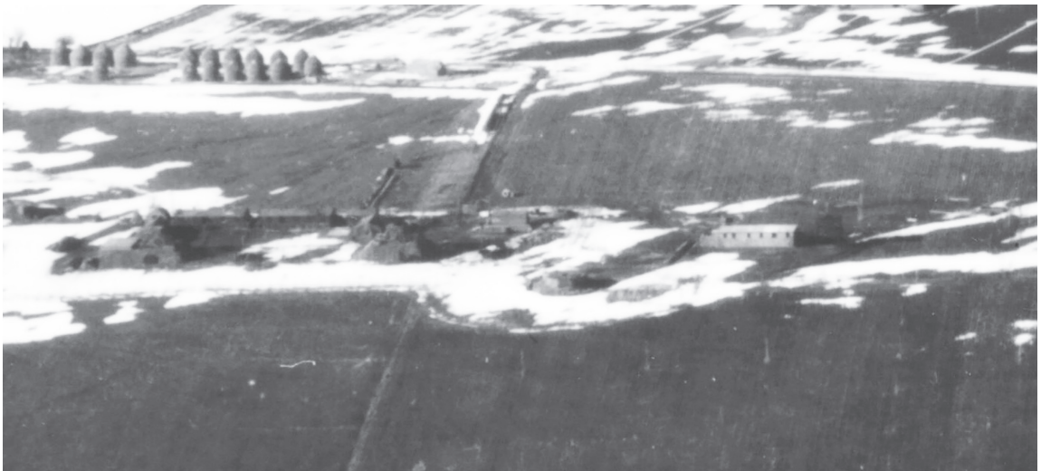
123 St Cyrus 1941 Type CHL, with the combined T & R Block and 20 foot aerial gantry visible at centre right, taken on 16 February 1942.
