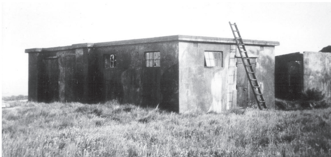
152 Westburn CD/CHL T & R Block with the aerial array and gantry removed, taken in June 1948 as work started to convert the building into a house.
