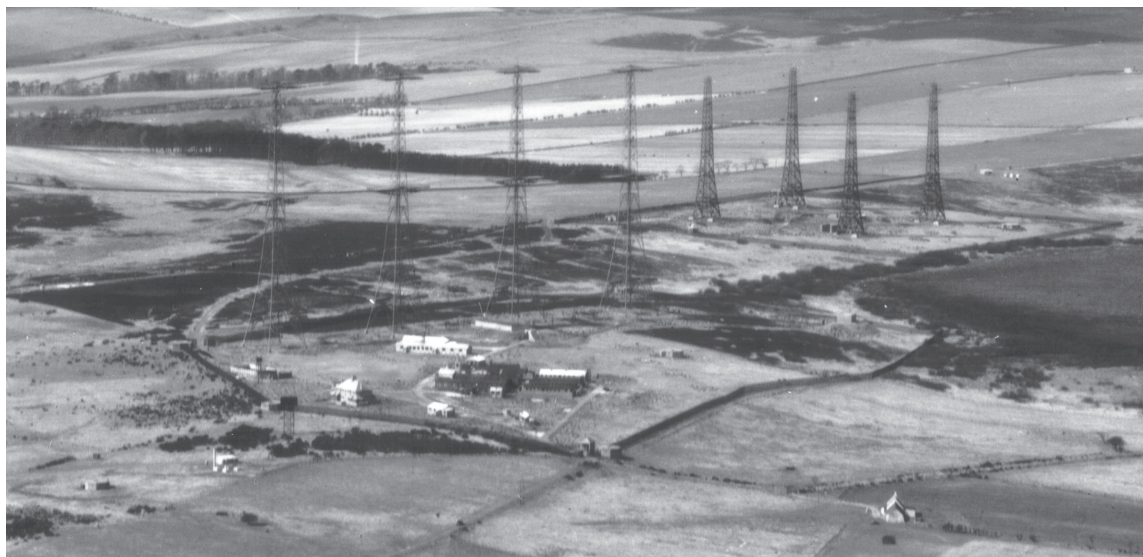
11 A typical East Coast type Final CH station, with the four 350 foot steel transmitter towers on the left and the four 240 foot wooden receiver towers on the right.
