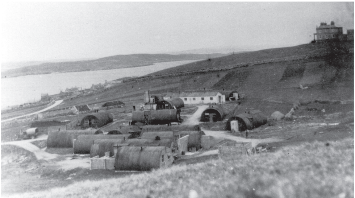
52 Clett Domestic Site, with Symbister House overlooking the site at the top right. (© Thomas Reid)
