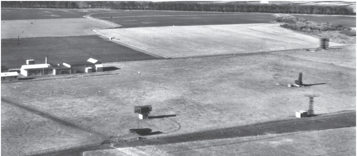
65 Dirleton GCI, photographed on 21 February 1950, with the Happidrome centre left, the Type 14 in the centre foreground (with the recently removed 'cheese' type aerial sitting on the ground in front), the IFF in the right foreground, the Type 13 behind it and the Type 7 in the top-right corner.
