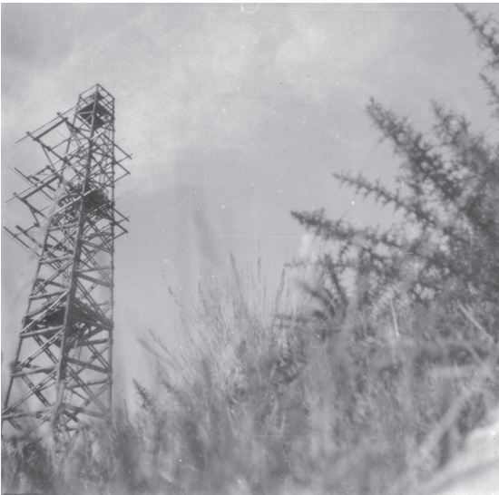
96 One of the receiver towers at Hillhead, showing the receiver dipole aerials mounted on supports from the tower.
