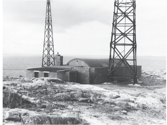
108 Mangersta, taken in 1956, showing the main technical building. (© Bill Smith)
