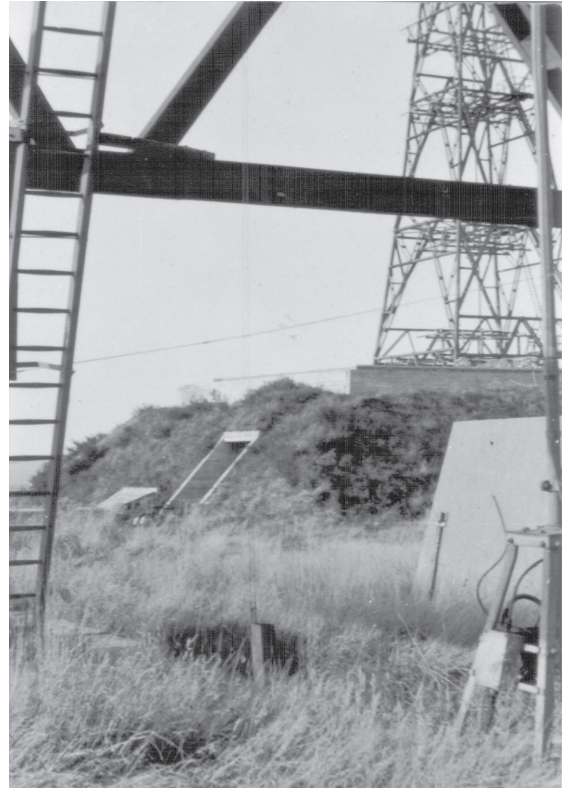
97 Hillhead Receiver Block with a receiver tower behind, taken from underneath one of the receiver towers.
