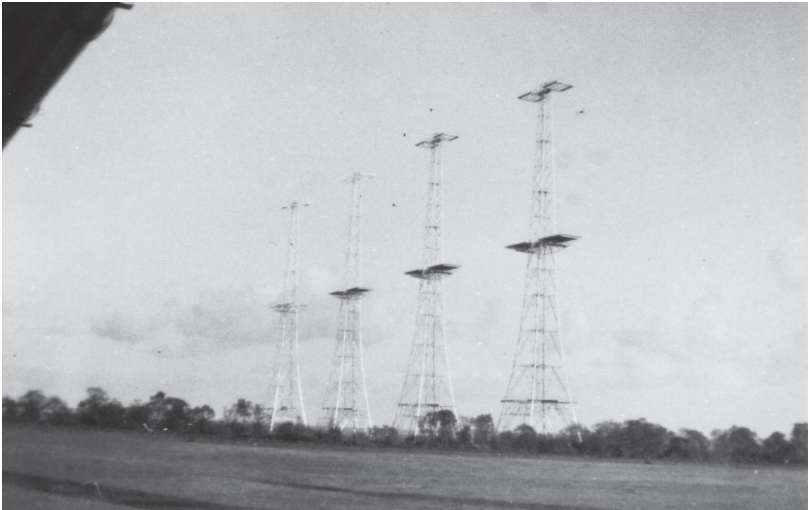
67 Douglas Wood in 1939 with the Final CH transmitter towers almost complete (note the far tower lacks wood on the middle platform).
