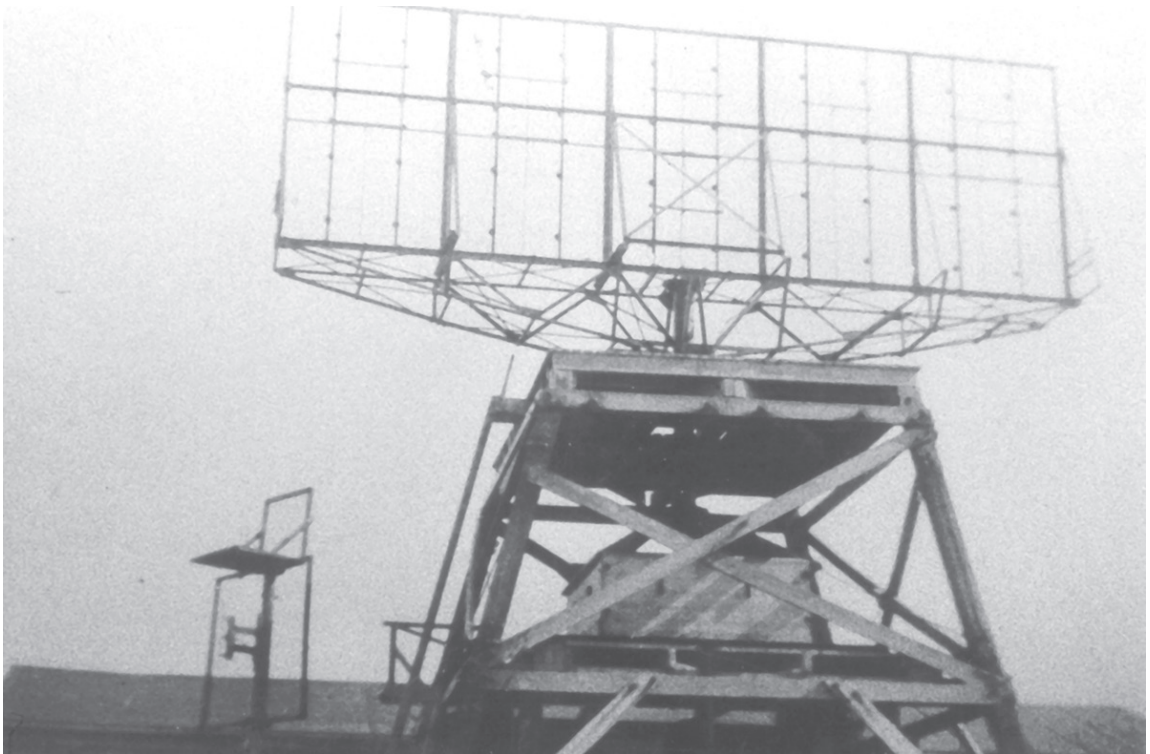
99 The CHL gantry and aerial array at Islivig, taken in 1946 when the station was on care and maintenance. (© Jim Russell)
