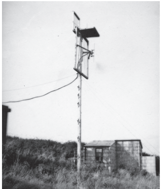
40 A pole-mounted aerial system for IFF Mk III at CHL stations.
