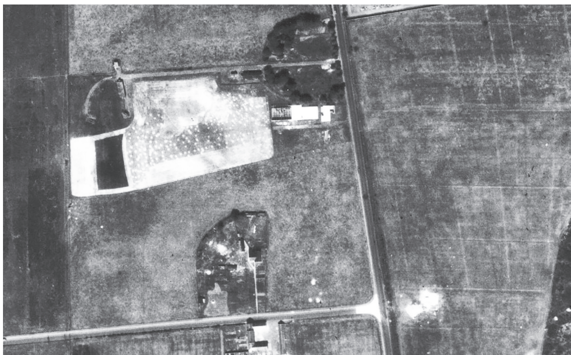
88 Vertical aerial photograph of Fullarton, taken on 1 August 1945, showing the Happidrome at upper centre as a white shape. Note the main operations room on the left side is not roofed, indicating clearly that the building is unfinished.
