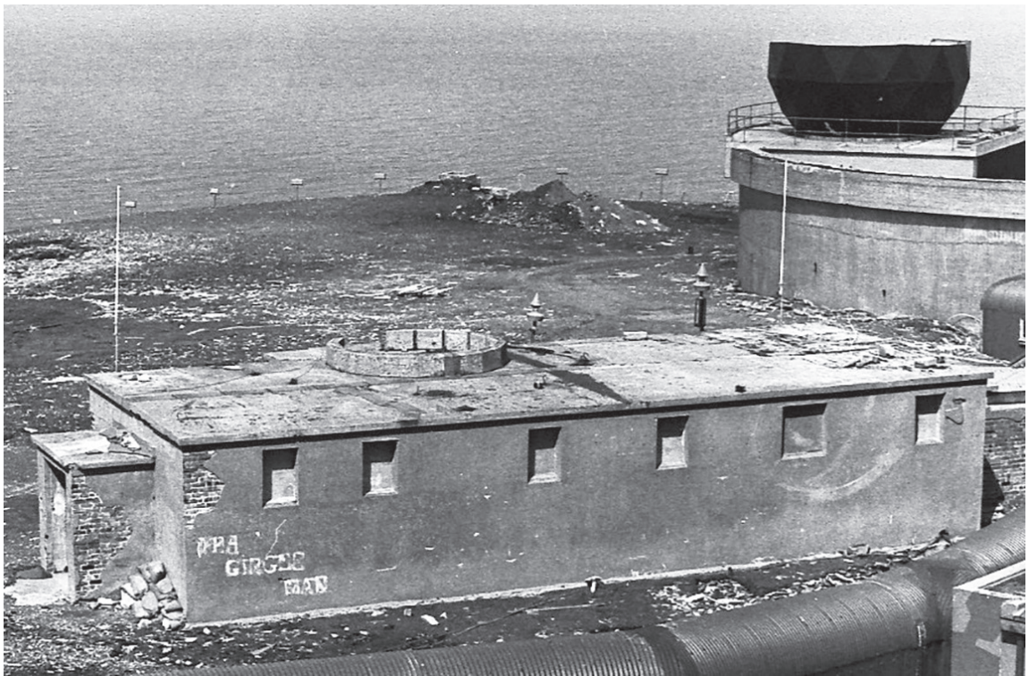
133 The combined T & R Block, taken in 1983, showing the location of the circular lantern for the Naval Type 273 paraboloids. This required a slight extension to the side of the building which is just visible behind.
