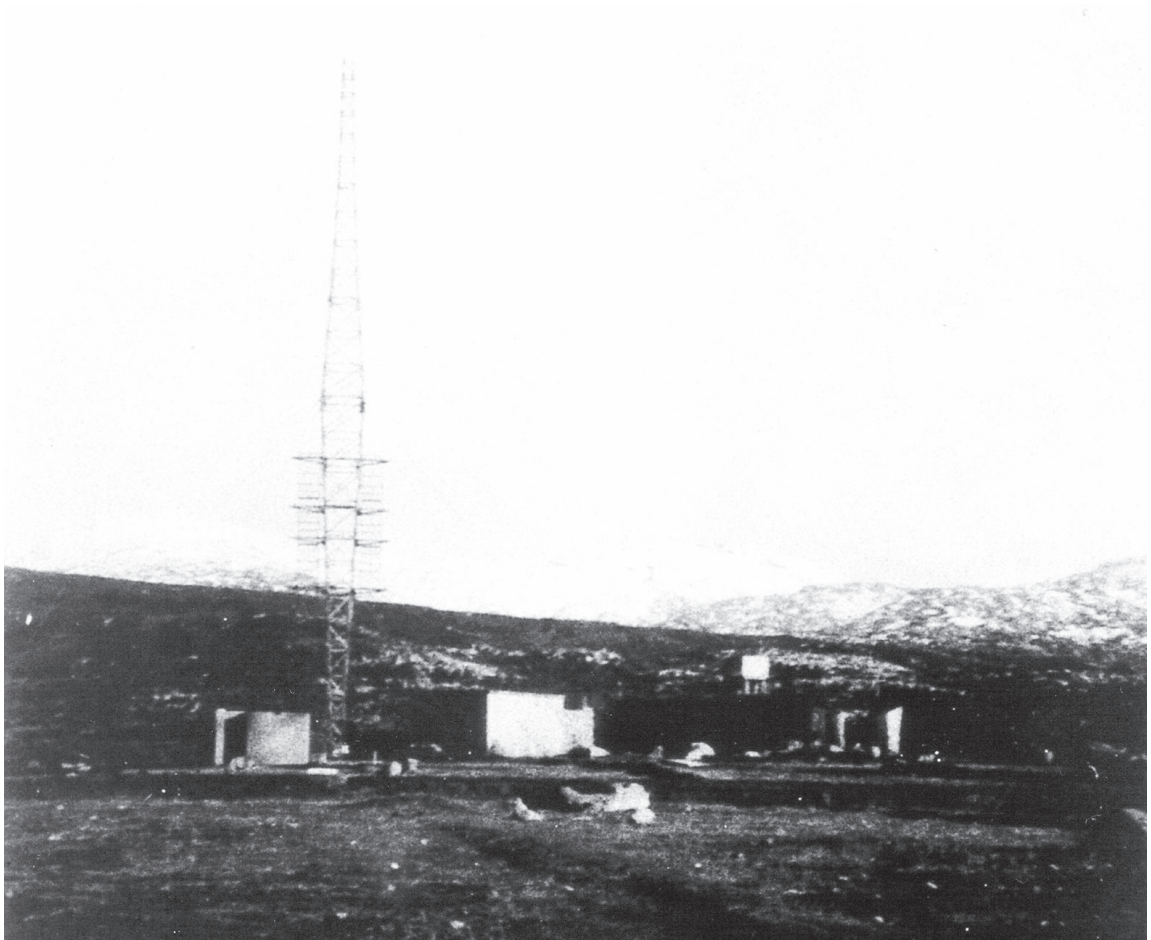
45 The IFF Mk III mast and building at Brenish on care and maintenance in 1946.
