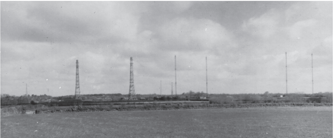
14 A typical West Coast type Final CH station, with the two 240 foot receiver towers at centre left and the four 325 foot transmitter masts in the centre and right of the photograph.
