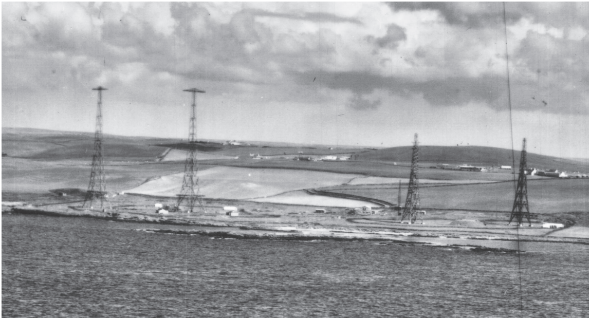
115 North Cairn from the air on 25 May 1948, showing the two 350 foot transmitter towers on the left and the two 240 foot receiver towers on the right, with the IFF mast just visible to the left of the receiver towers.
