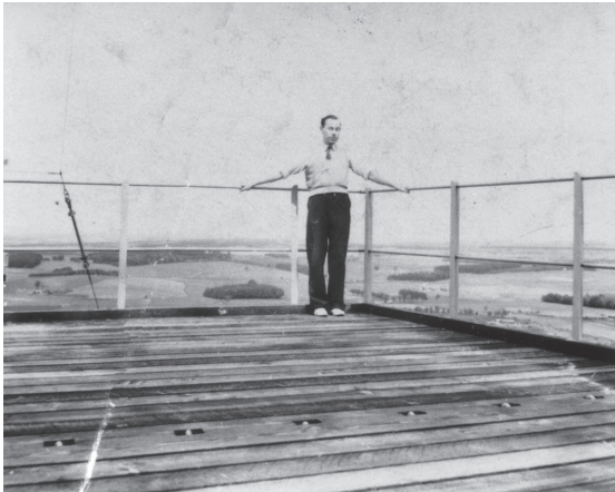
68 Alex Hunter on the 200 foot platform of one of the transmitter towers at Douglas Wood. (© Alex Hunter)
