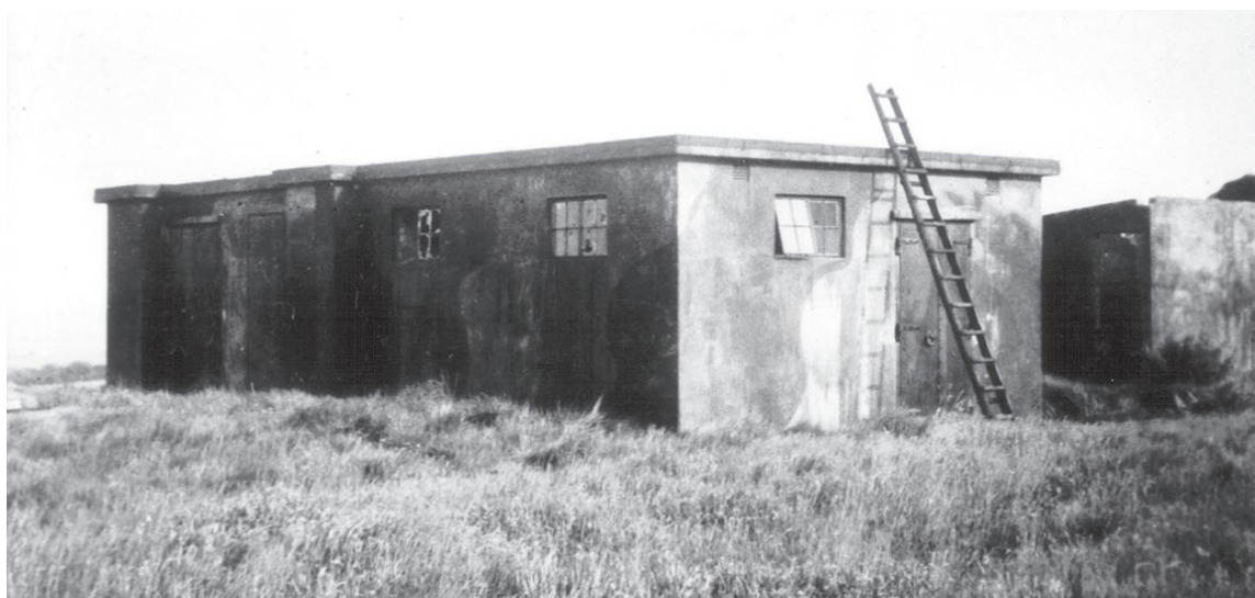
152 Westburn CD/CHL T & R Block with the aerial array and gantry removed, taken in June 1948 as work started to convert the building into a house.
