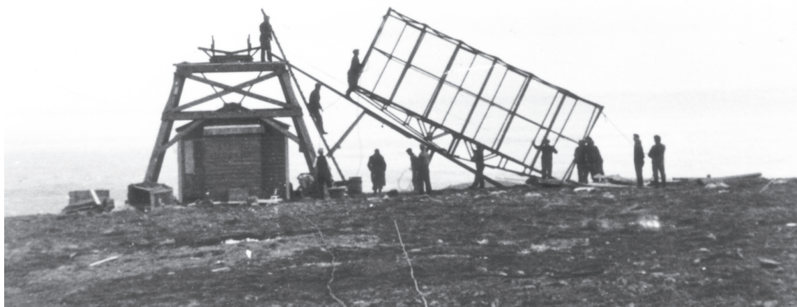
82 Erecting the aerial frame, all done by block and tackle, planks and manpower, at Fair Isle North Transmitter Hut, early 1940.
