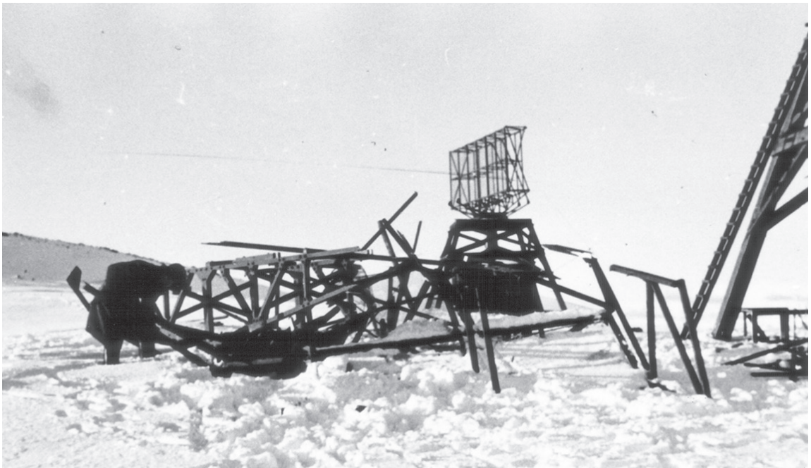
84 Fair Isle North (AES 2) showing the results of gale damage in January 1940.
