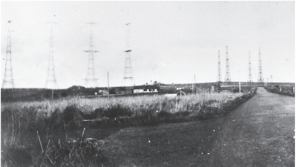
112 Netherbutton, with the four 350 foot transmitter towers on the left and the four 240 foot receiver towers on the right.
