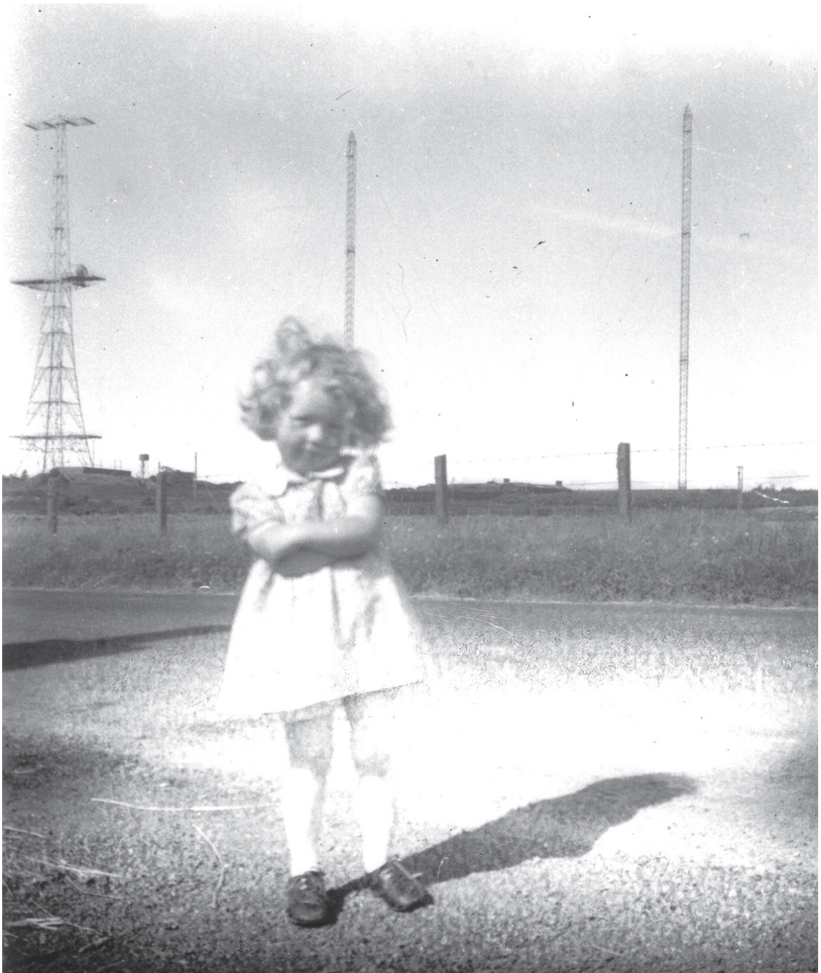
71 One of the 350 foot transmitter towers at Douglas Wood, with the two 325 foot guyed transmitter masts which replaced the two removed towers. Note the Type 55 radar on the 200 foot platform of the tower.
