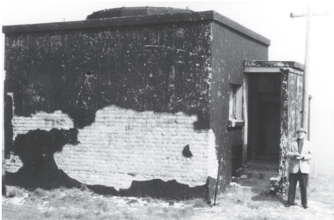
76 Transmitter Hut of the CDU station at Dunnet Head, photographed in June 1965. Note the ring on the roof for the Perspex lantern which housed the Naval Type 273 radar paraboloids.
