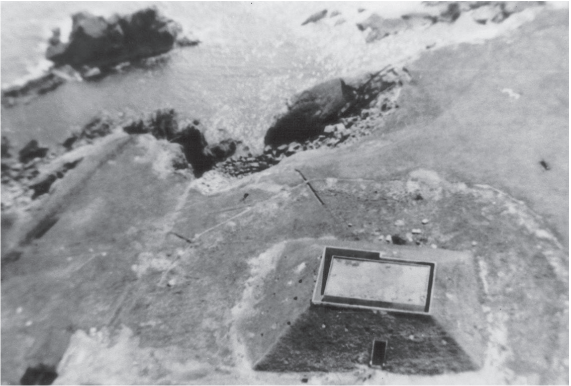
139 Skaw Stand-by Set House, the back-up power station for the site, taken in 1947.
