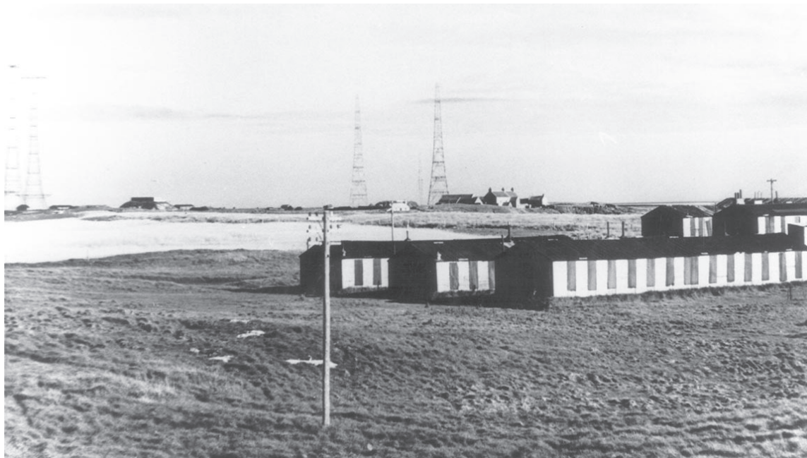
153 Whale Head from the Domestic Site, showing the two 350 foot transmitter towers on the left, the two 240 foot receiver towers in the centre and the 105 foot IFF mast next to the right-hand receiver tower. (© Kenny Foubister Collection)
