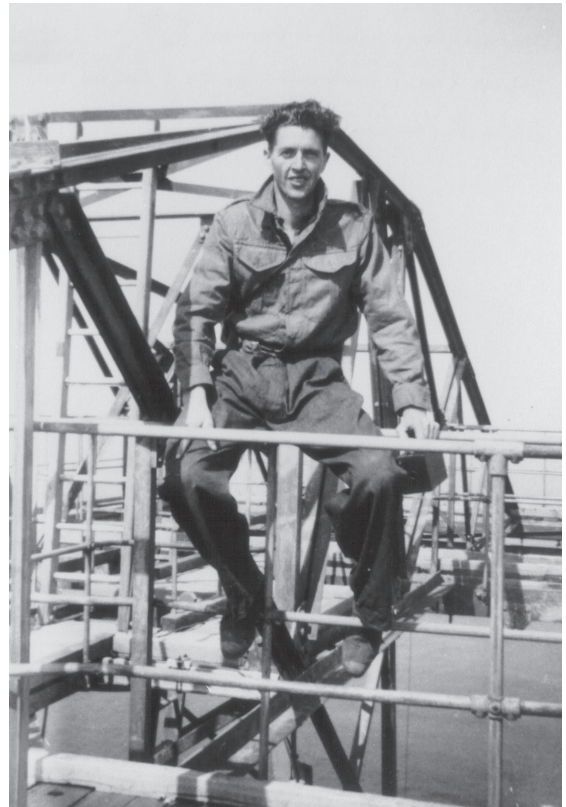
137 Andrew Laurenson at the top of one of the 350 foot steel transmitter towers at Skaw in 1947. (© Andrew Laurenson, via Leslie Smith)
