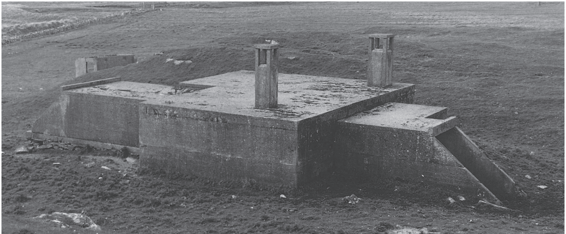
15 Type C Transmitter Block at Saligo, taken in 1996. (© Historical Radar Archive)
