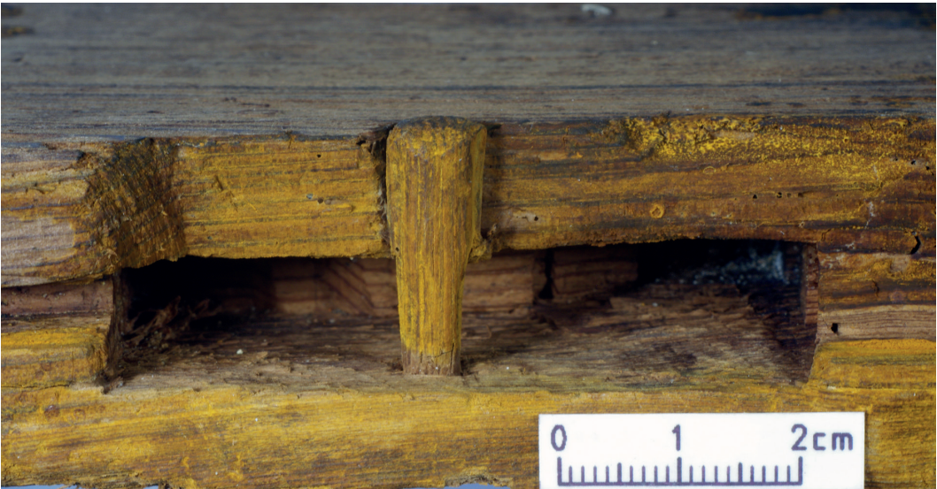
Illustration 153 Joint in moulded panel frame [26]
