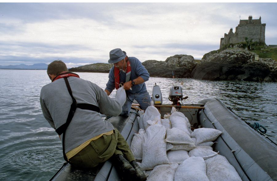
Illustration 26 Sandbags filled with gravel being delivered to the site (Edward Martin, DP 174780)
