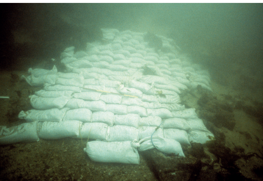
Illustration 27 Sandbags freshly laid over an exposed organic deposit (DP 174786)
