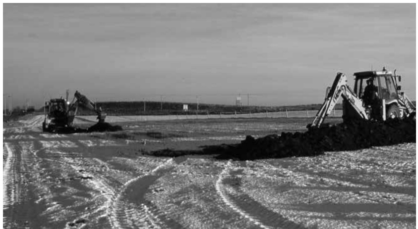
1.2 Evaluation of the road corridor underway, winter 2002.
