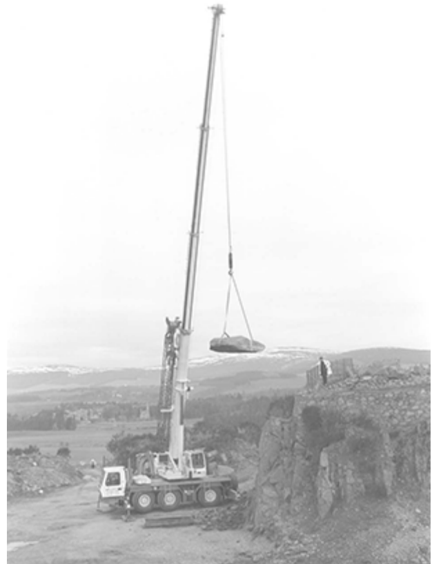
40 Lifting one of the displaced flankers at Tomnaverie.
