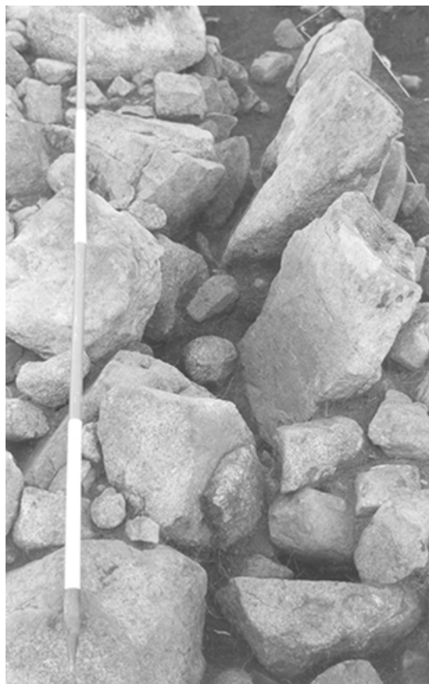
23 Packing for the displaced kerb at Tomnaverie, showing how it had been wedged in position in between two masses of rubble.
