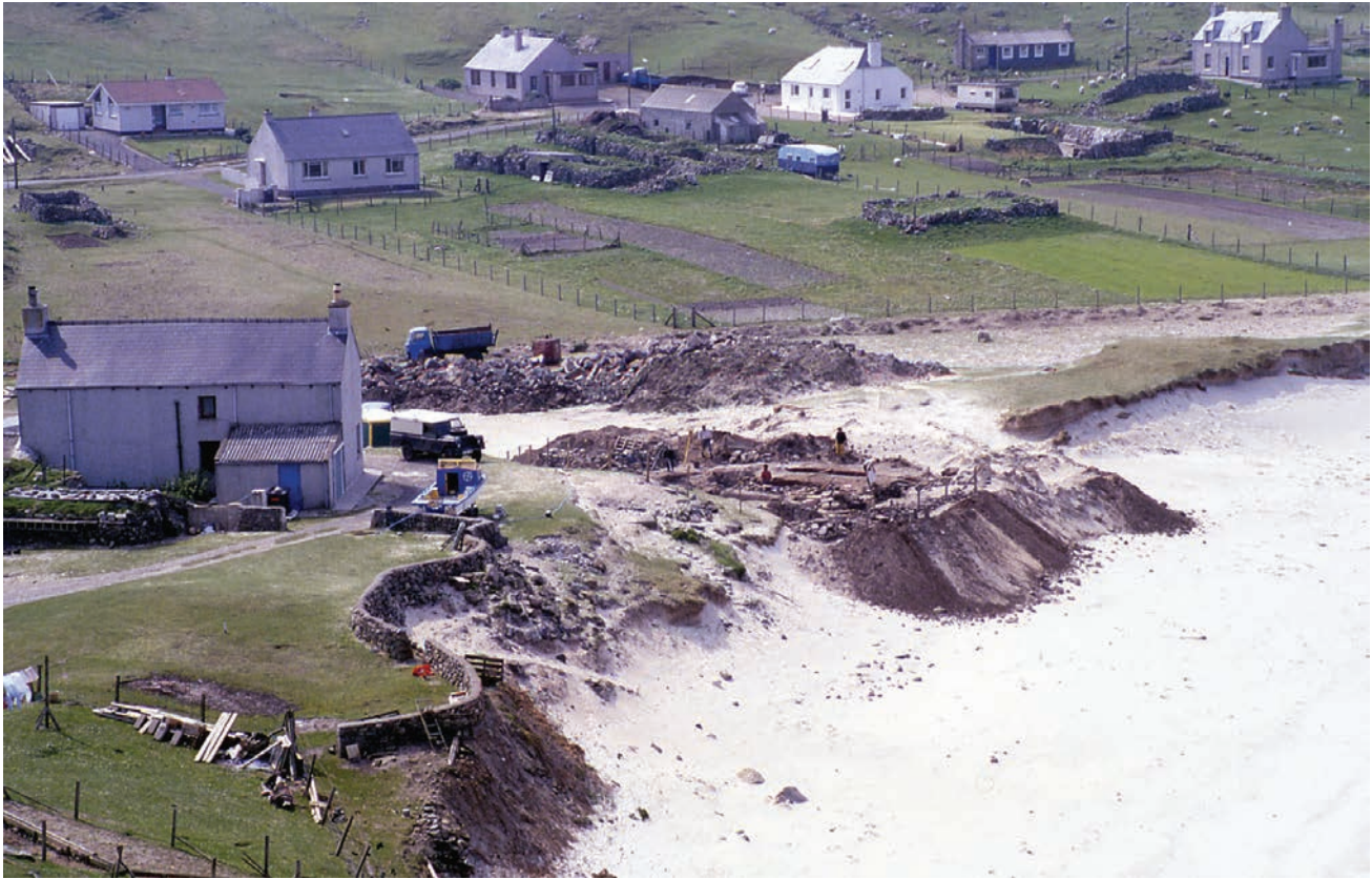
1. The excavations in progress
