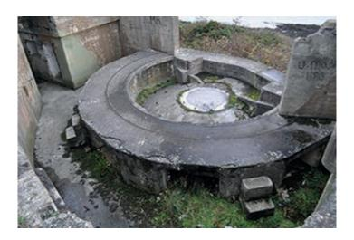
The 6-pdr emplacement at Charles Hill. The canopy over the rear of the emplacement has been removed (© Gordon Barclay)
