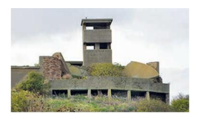
Figure 10.17 The southern 6-pdr twin gun-house, incorporating the southernmost 4-inch emplacement, and built out upon concrete pillars, with the Director Tower behind (© Gordon Barclay)
