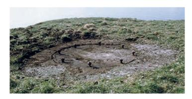
Figure 10.38 The large hold-fast (eight bolts in a circle c 1.5m in diameter) near the western end of Inchcolm, for the First World War 3-inch anti-aircraft gun. This photograph was taken in the 1980s (© Ron Morris)
