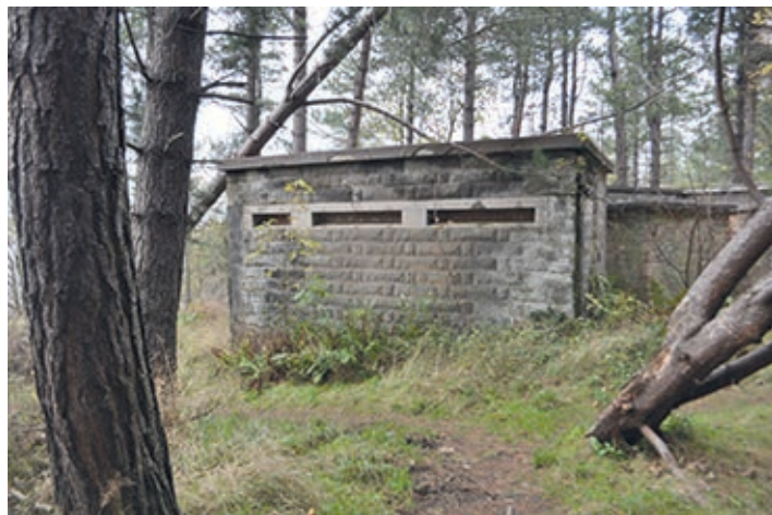
Figure 10.44 The loop-holed western end of the barrack block (© Gordon Barclay)
