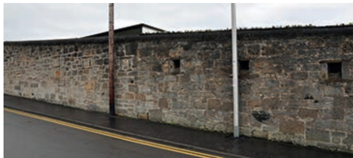
Figure 11.73 Surviving portion of the loop-holed boundary wall on Pettycur Road (© Gordon Barclay)
