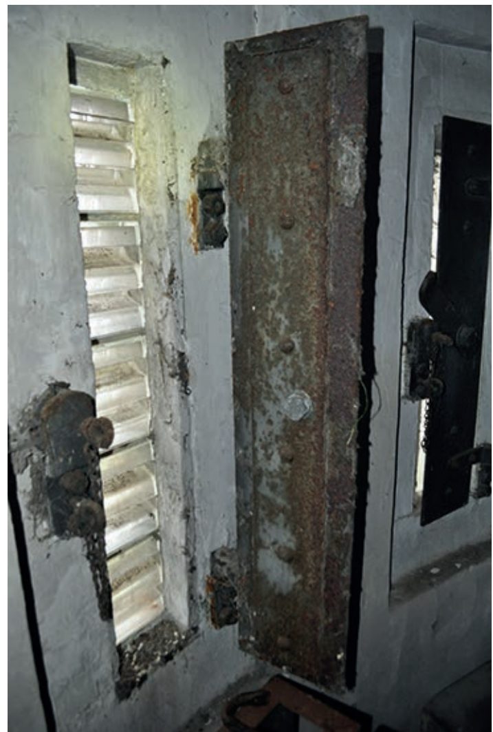
Figure 10.37 DEL emplacement No. 3 on Inchcolm, with its central prism-filled window and its internal steel shutter (© Gordon Barclay)
